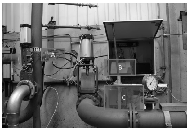
Figure 2. Measurement system installation at the full-scale industrial biogas plant. (A) MIR Probe, (B) MIR Spectrometer, (C) UNICAL cleaning system.
